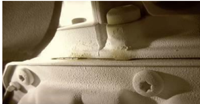
Figure 4. Leak located with talcum spray.
