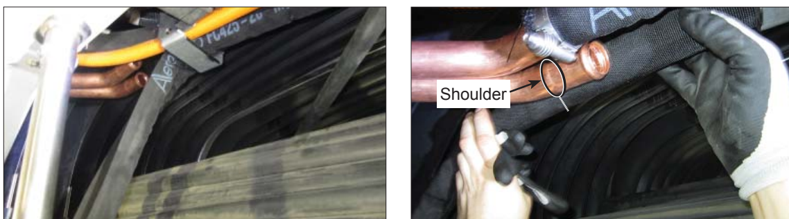
Figure 12 - Measure and Cut the Flexible Hoses
