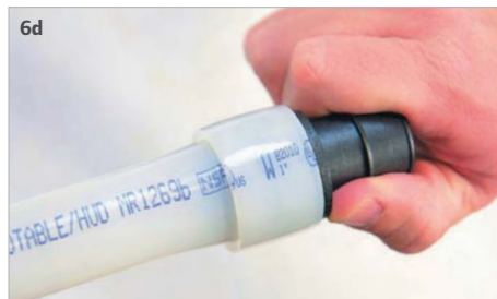
6d Insert ProPEX Fitting into 1" Uponor PEX Piping.
