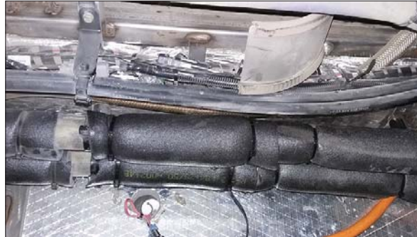
Figure 17 - Insulation on the Copper Pipes
