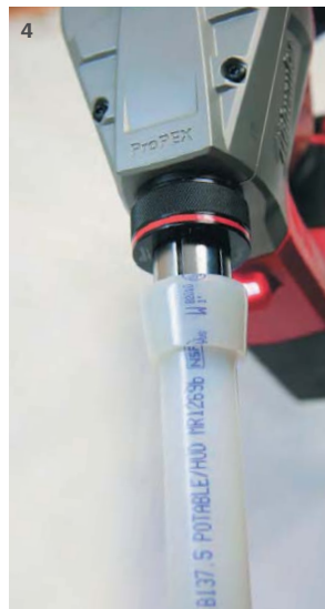
Expansion with Milwaukee M18 ProPEX Expansion Tool
