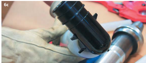
Insert ProPEX Fitting into 2" Udonor PEX Piping.
