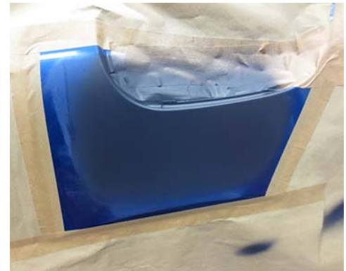
Surface primed and filled
