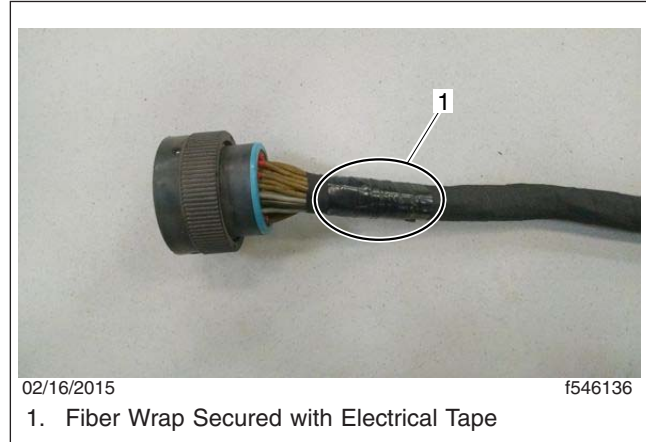
Fig. 15, Fiber Wrap Secured with Electrical Tape
