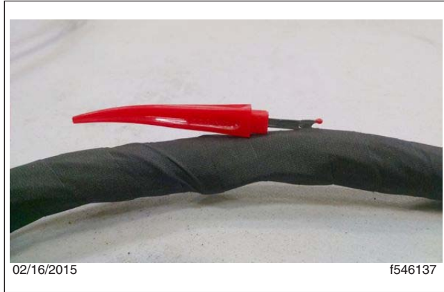
Fig. 9, Cutting an Opening into the Fiber Wrap
