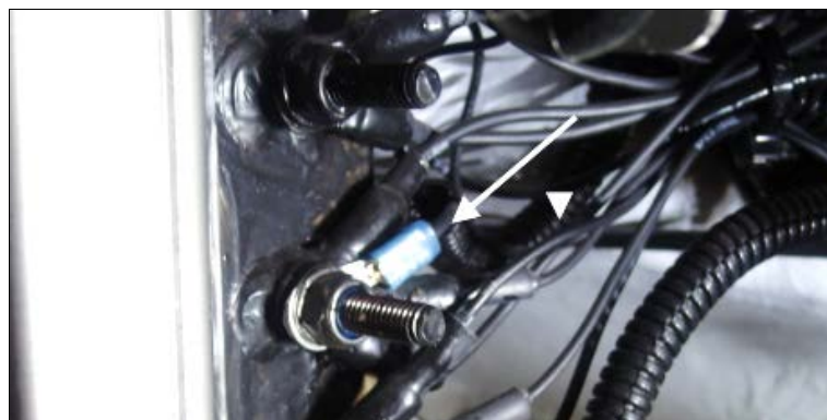
GROUND WIRE CONNECTED
