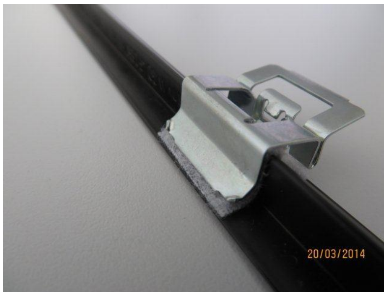
Figure 4. Retaining clip isolated with the fleece adhesive tape.
