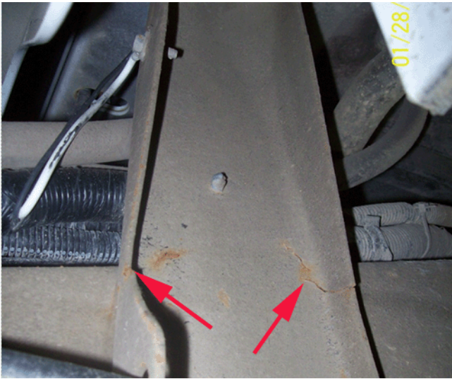
Example of mounting bracket with cracks developing (not all mounting points used).
