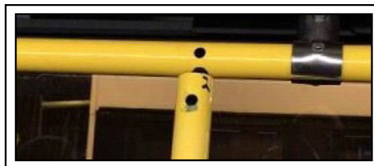
Figure 10 - Typical View of Wiring Slack
