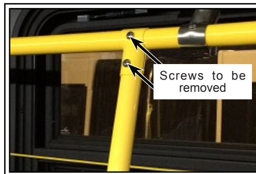
Figure 9 - Removal of Screws on the Stanchion
