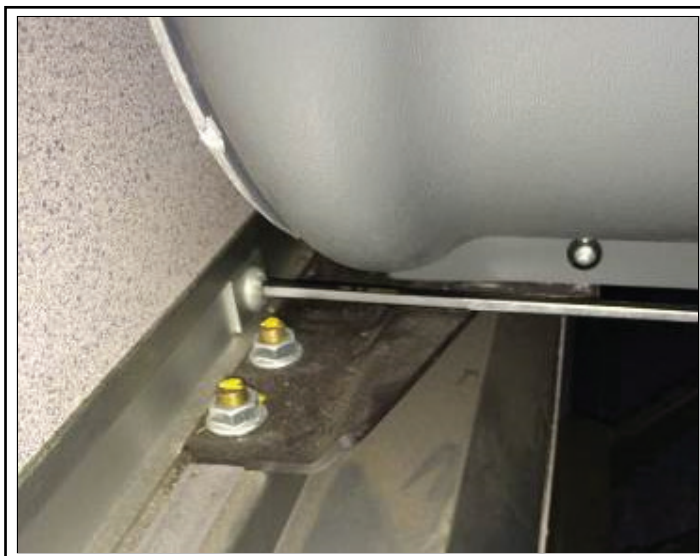
Figure 23 - Installation of Damaged Hardware to attach Seat Rail on Wall
