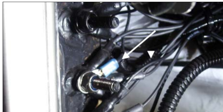
GROUND WIRE CONNECTED
