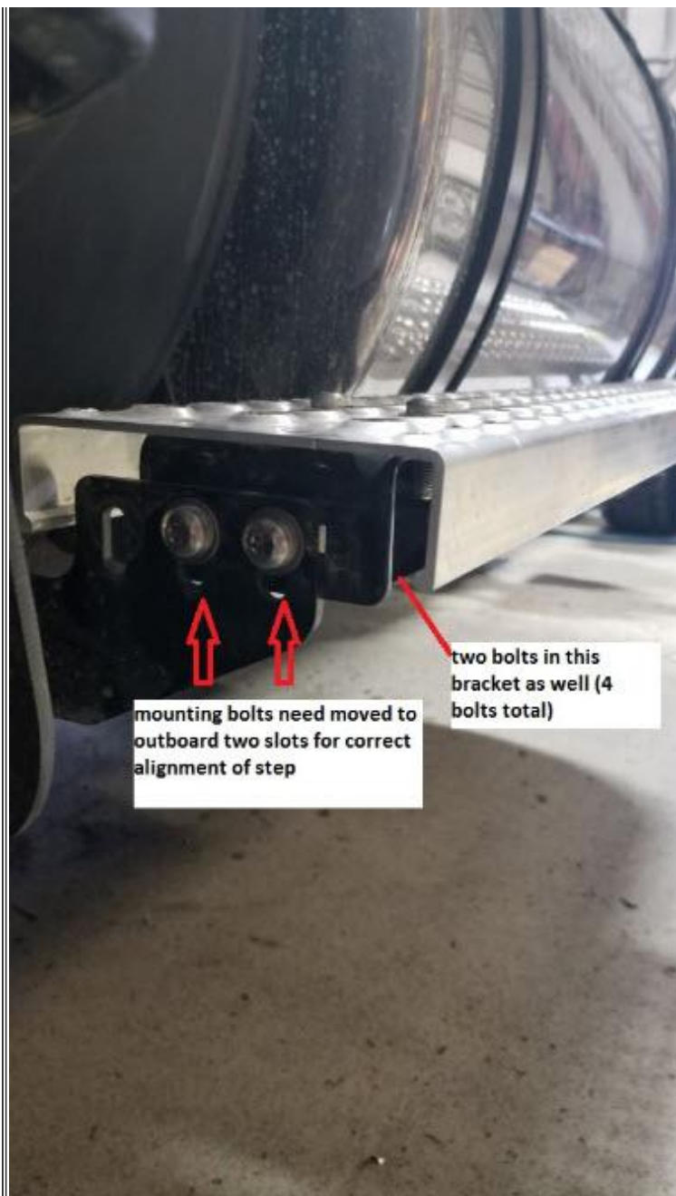
Figure 3: Bolts installed in the proper location
