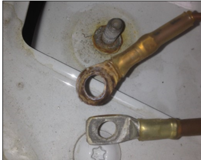
Figure 2 – Example of corrosion on ground point
