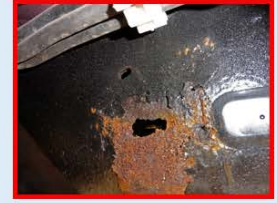
Perforation of the Frame
