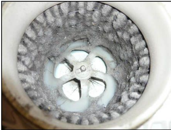
Figure 1. HV Battery Cooling Fan Before Cleaning
