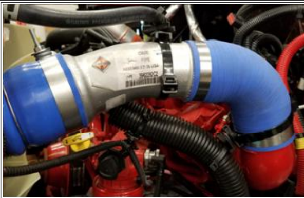
Figure 5: New CAC piping installed
