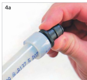
Insert ProPEX Fitting into Uponor PEX Piping.
