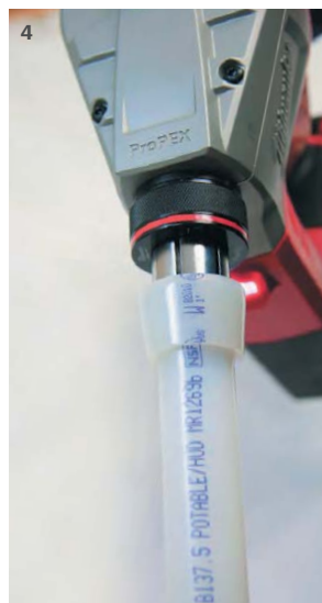
Expansion with Milwaukee M18 ProPEX Expansion Tool
