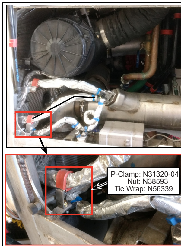
Figure 12 - Installation of P-Clamp and Tie Wrap
