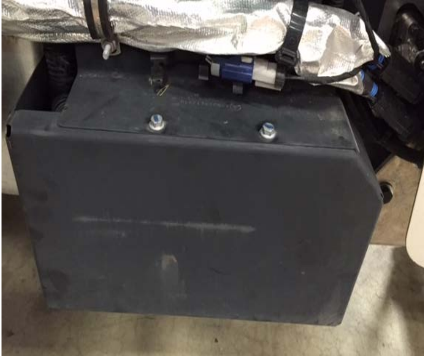
Figure 14 – ACM Cover Installation
