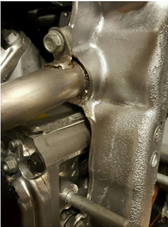
Coolant leak at the O-ring seal of the Exhaust Gas Recirculation (EGR) coolant feed pipe. Refer to call out #2 in the above picture.
