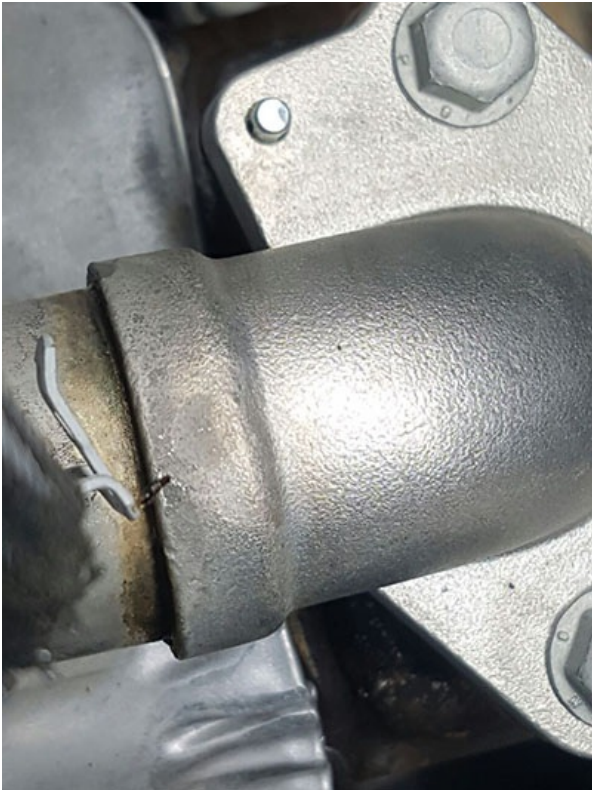
Welded flange leaking on the Exhaust Gas Recirculation (EGR) coolant feed pipe. Refer to call out #2 in the above picture.
