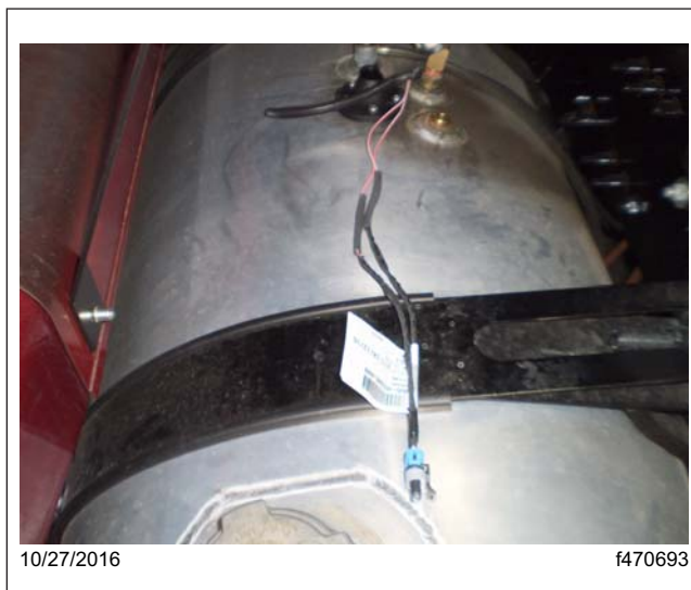
Fig. 9, New Pigtail Installation
