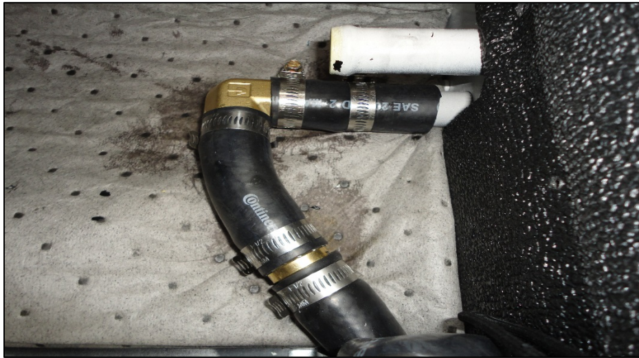
Figure 10, Installation of 4 inch lines onto elbow
