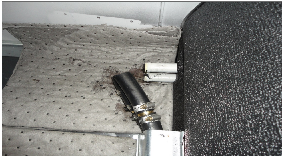
Figure 7, Installation of 4 inch hose and brass fittings
