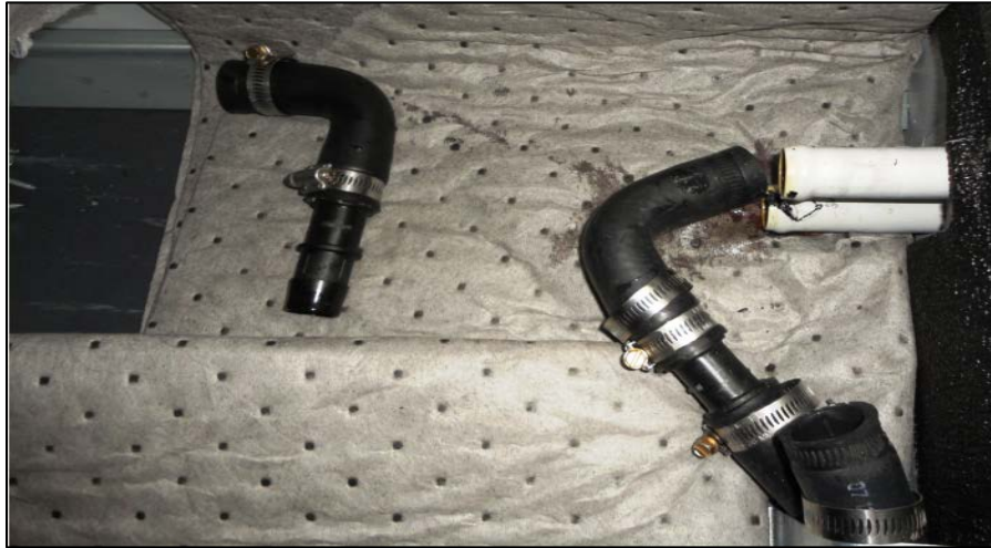
Figure 6, Removal of rubber elbow
