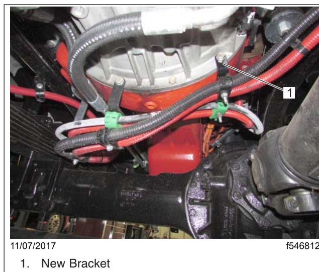
Fig. 5, New Battery Cable Installation
