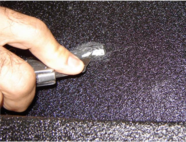
1. Use a utility knife or screwdriver to remove any loose debris from the repair area. Bevel the edge of the repair area with the utility knife.
