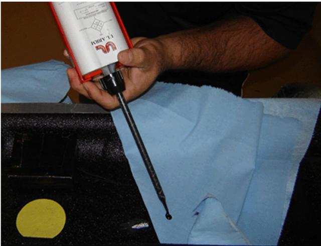
5. Purge the mixing tip away from the repair area (on the towel) to ensure proper material mix. Pump the cartridge at least 3 times verifying there are no striations in the material to ensure proper mix. The material should be a solid black color.
