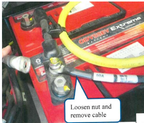
Figure 21: 2/0 CABLE REMOVAL FOR 4/0 RECONNECTION
