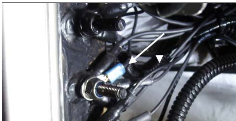
GROUND WIRE CONNECTED
