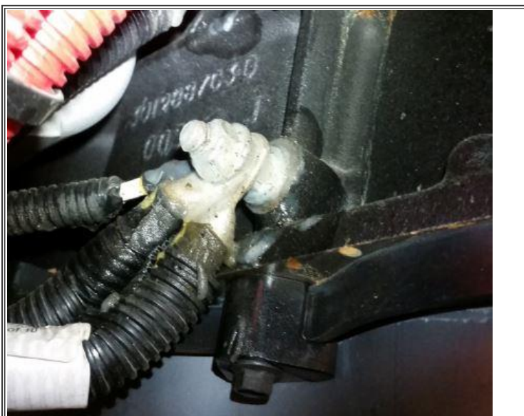
Figure 1: Ground cable connection
