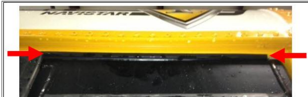
Upper Door Casing Seal Evenly Compressed
