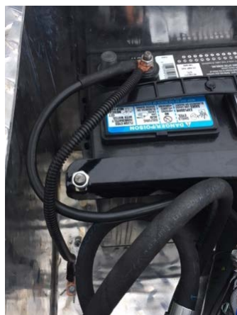
Completed Repair - With Ground Wire
