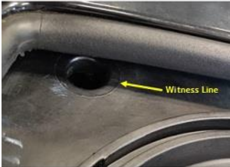
Figure 15 Drain hole and witness line.
