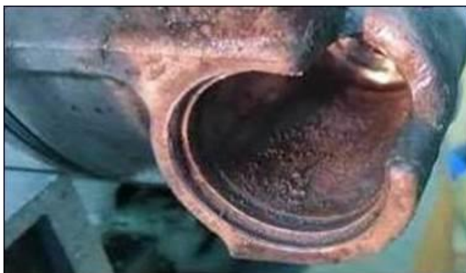
Figure 14. Corrosion in the N280 valve bore.
