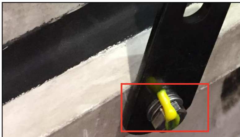
Figure 9 - Torque Seal Application
