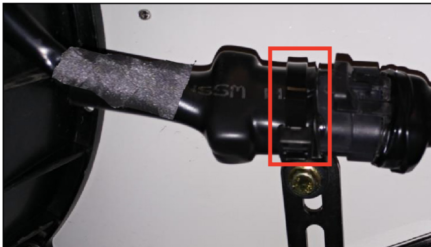
Figure 14 - Cable Tie (G5007995) Installation
