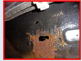
Perforation of the Frame
