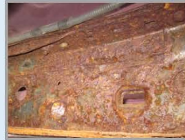
Complete Surface Rust with Descaling
