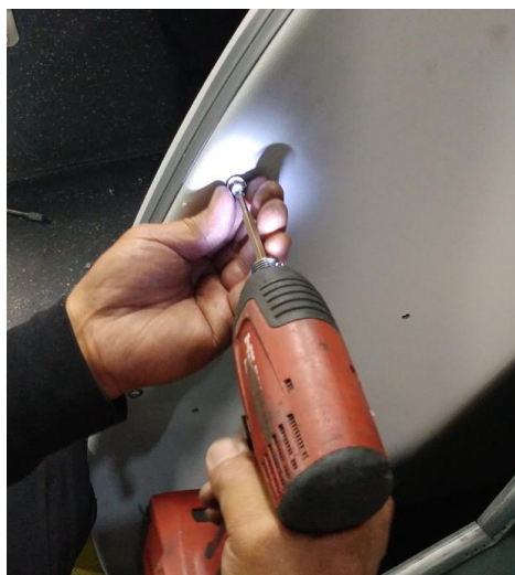
Figure 14: Secure Panel Caps in Place
