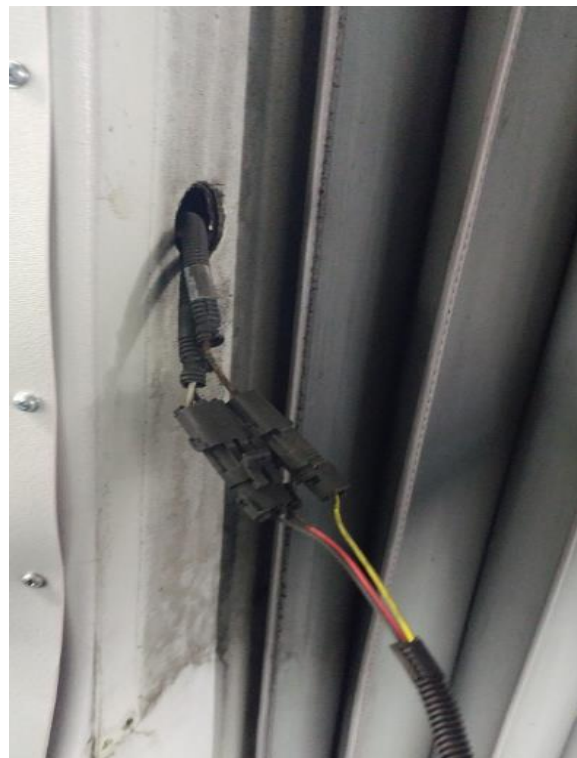
Figure 3: Remove Artic Joint Lights
