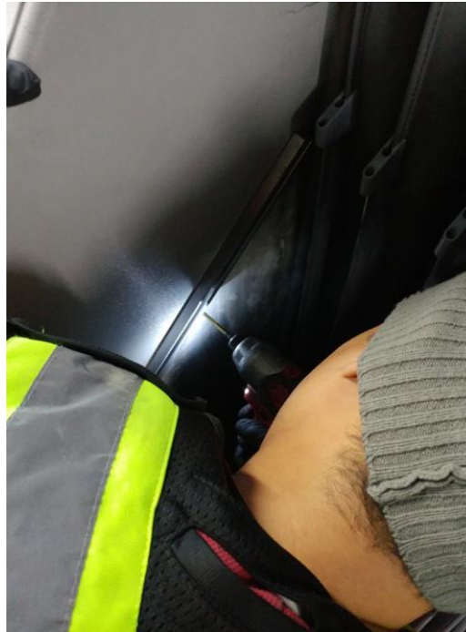
Figure 7: Drill out Rivets
