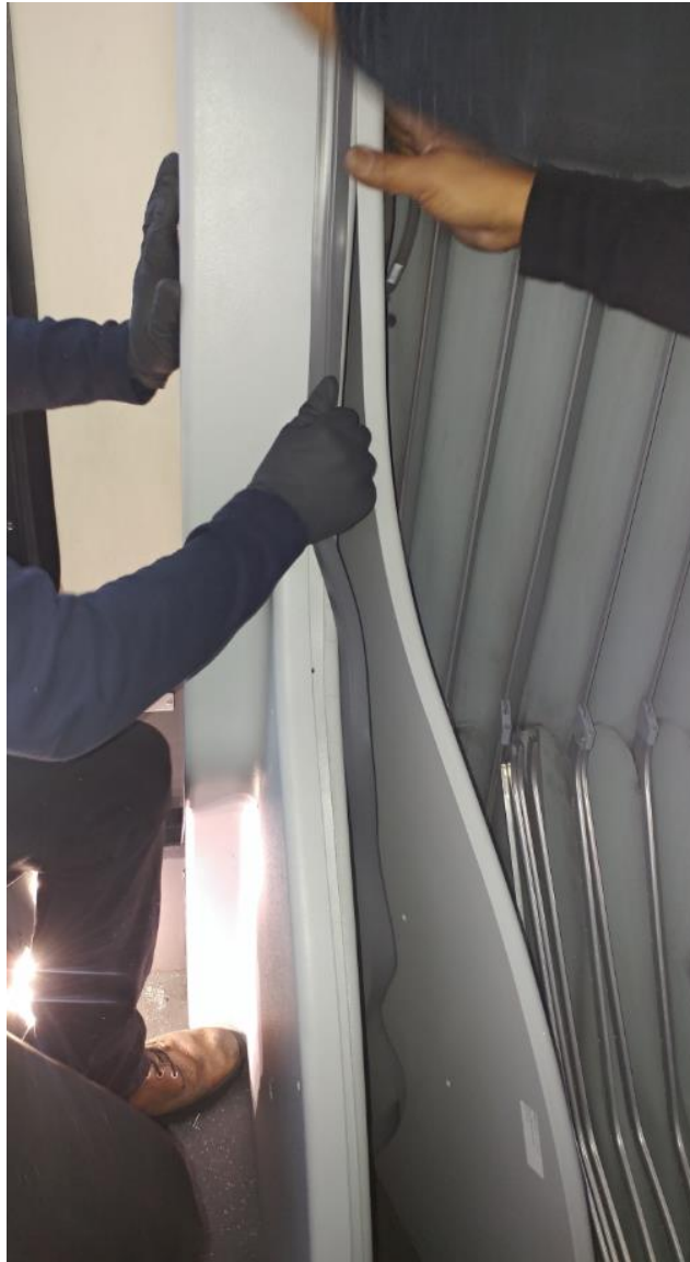
Figure 12: Install H-Channel
