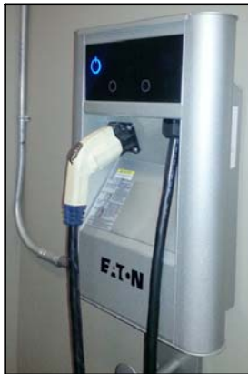
Level 2 Charging: 240V Charging Station (Eaton shown as example)
