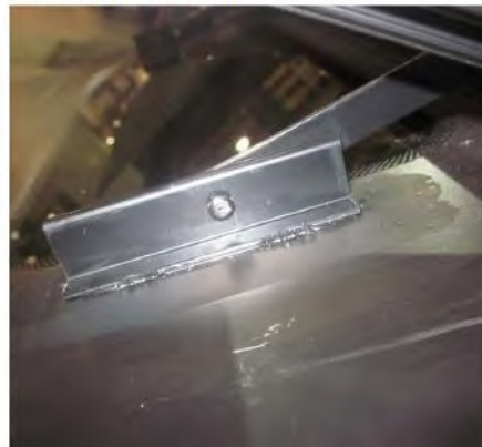
STEP 4. RIVET INSTALLED
