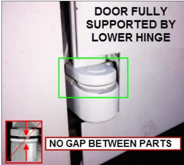
FIG.6 LOWER HINGE SUPPORT
