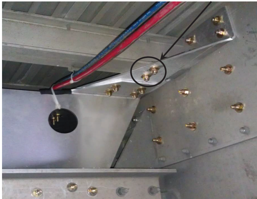
Figure 3. 40106506 bolted at cross-members
