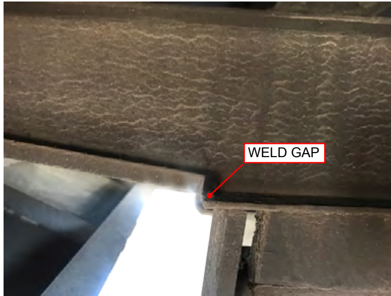
Overview of weld reinforcement repair
