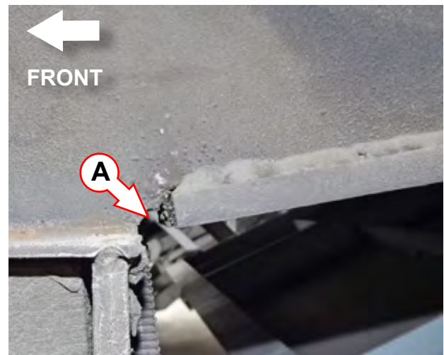
Incomplete weld (A) at LH long sill
