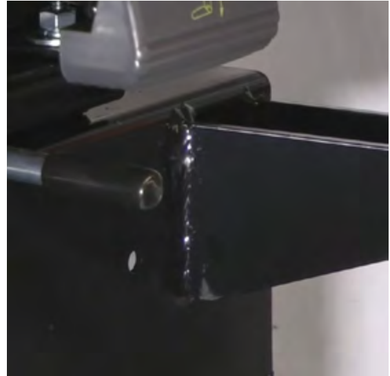
An example of a good continuous weld
