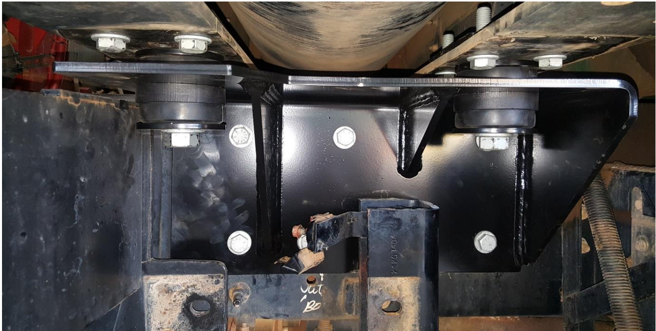
Figure 15. New bracket, bolts and isolator properly installed.
