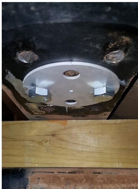
Figure 8. Place the drill template (round disk) as shown, bolt it into place and drill a new 3/16-in. pilot hole in the center for the isolator. Then, remove the drill guide and ream the center hole to 15/16-in.
