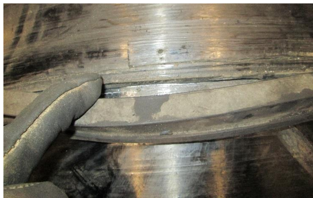
Figure 3. Isolator rib splitting away from the isolator channel.
