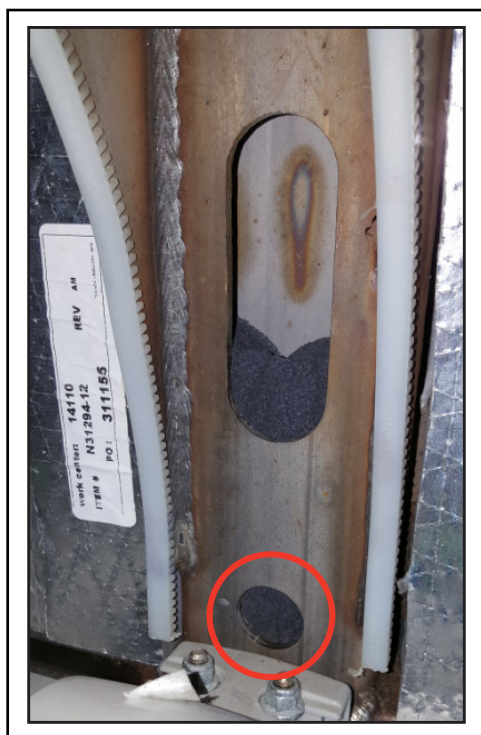
Figure 7 - Typical View of Hole and Cut-out covered with the Large Foam Piece
