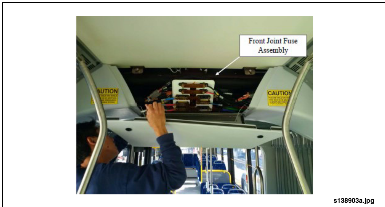
Fig. 1: Wiring Joint Fuse Assembly
