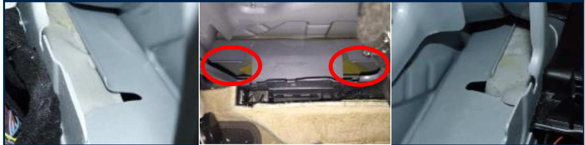
Foam piece installed
