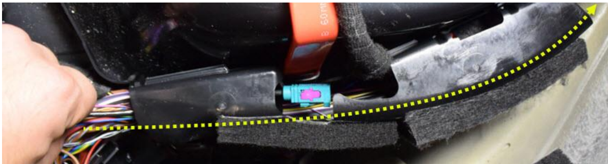
Figure 10. There is enough room inside the plastic conduit to feed the wire without opening it.
