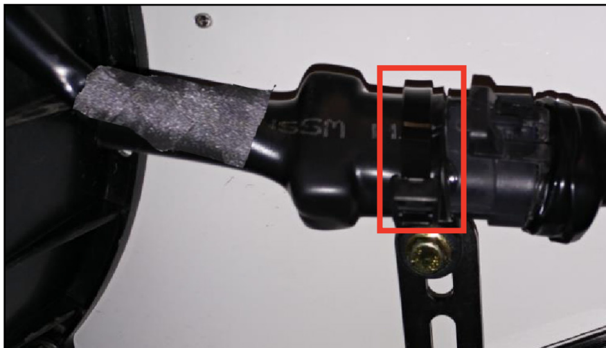
Figure 14 - Cable Tie (G5007995) Installation
