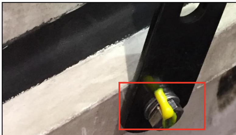
Figure 9 - Torque Seal Application
