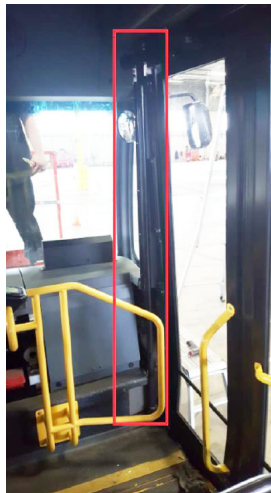
Figure 39 - Install the Front Right Door Post Capping
