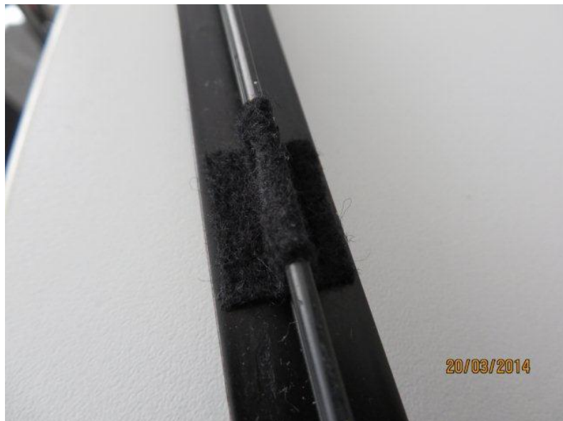
Figure 3. Fleece tape section applied.
